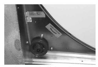
FIGURE 30: Wheel belt & pulley
